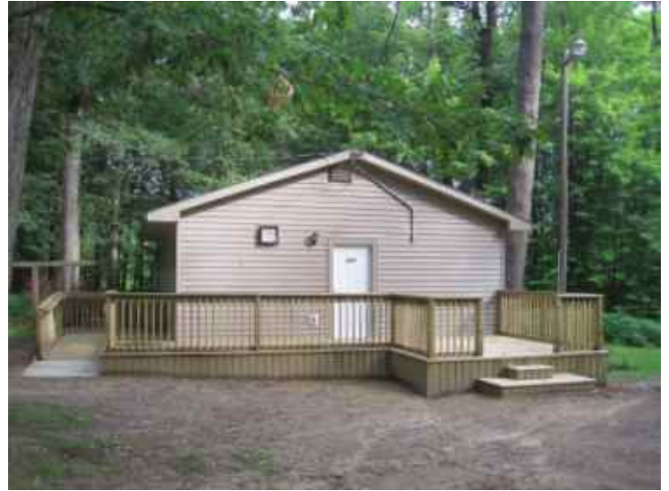
All the main Research and Education Centre buildings now meet Ontario Disability Access standards
